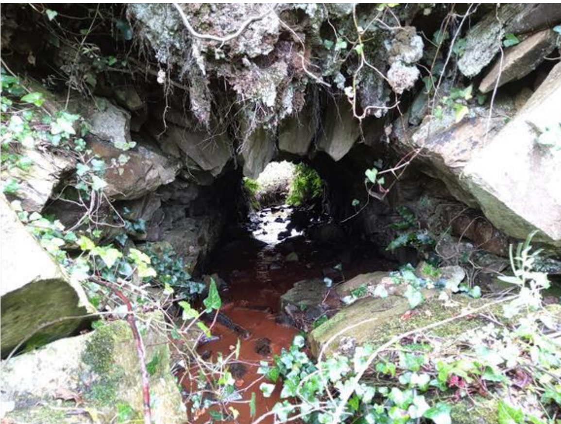
Collapsed sections of masonry arch
